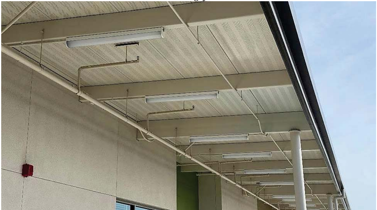
Figure 19. New Exterior Light Fixtures Installed in the 2nd Floor Corridor of the New Classroom Building for CO T-635
