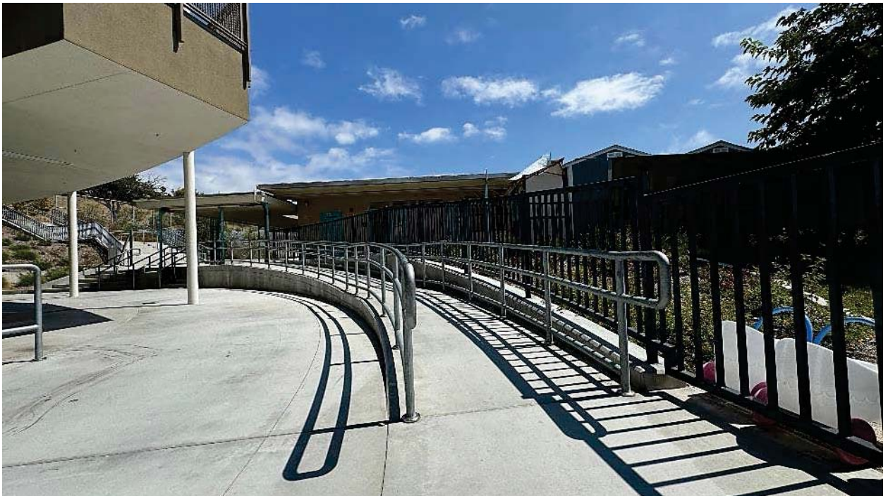
Figure 28. Accessible Path of Travel: New ADA Concrete Ramp
