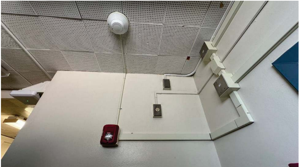
Figure 32. New Fire Alarm Devices and Wiremold Raceway Installed at MPR Building
