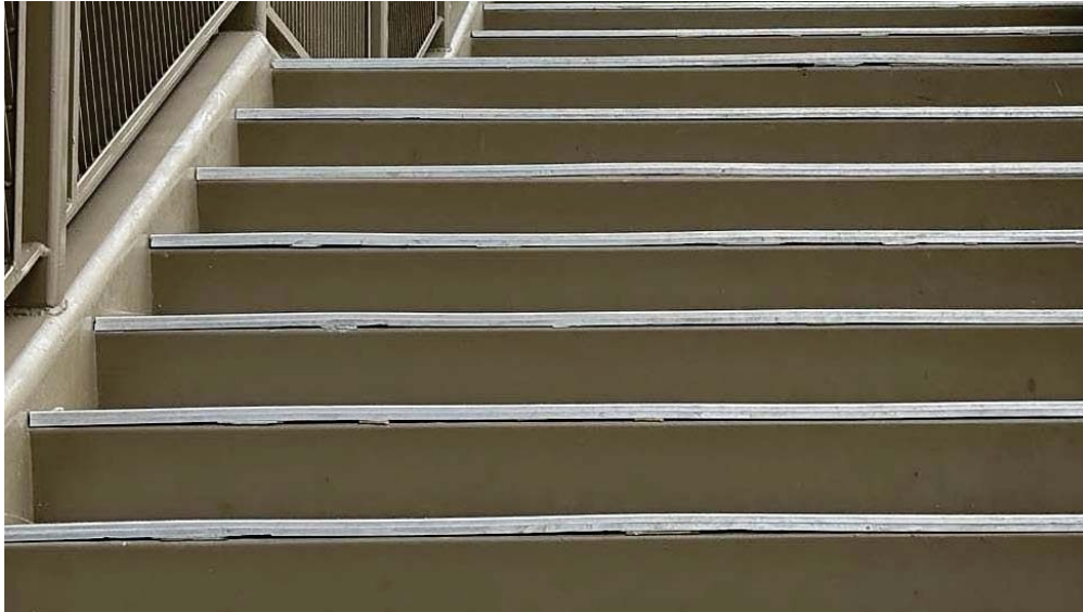
Figure 4. Visible Gaps between Stair Nosings and Treads in Stair 6-B
