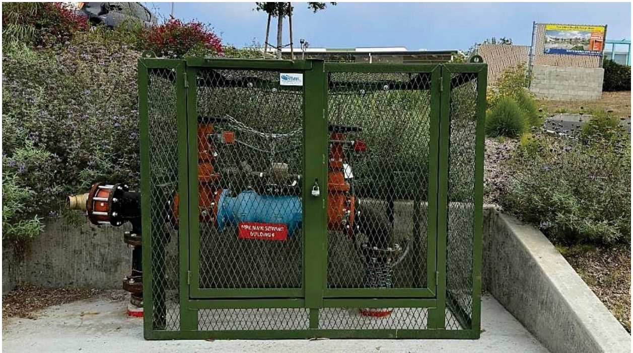
Figure 30. Double Check Detector Assembly
