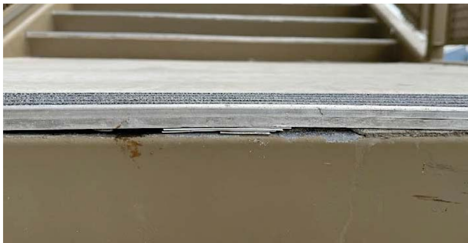
Figure 3. Close-up Photo - Visible Gap between a Stair Nosing and a Tread in Stair 6-A
