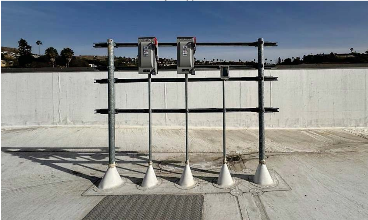
Figure 17. New Mounting Racks for Rooftop HVAC Disconnect Switches on the Classroom Building Roof for CO T-582
